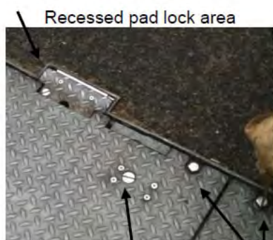
Hatch opening lock Hatch bolts
