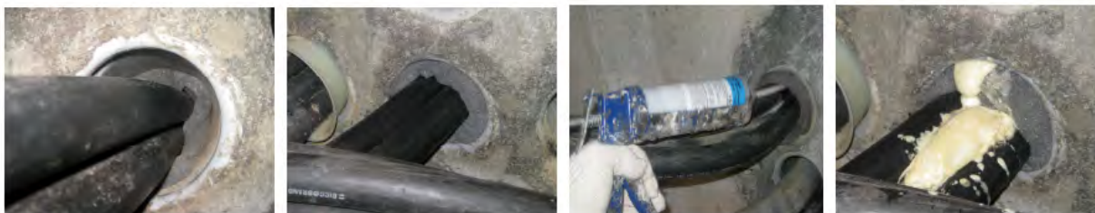
Water stop sealant installation
