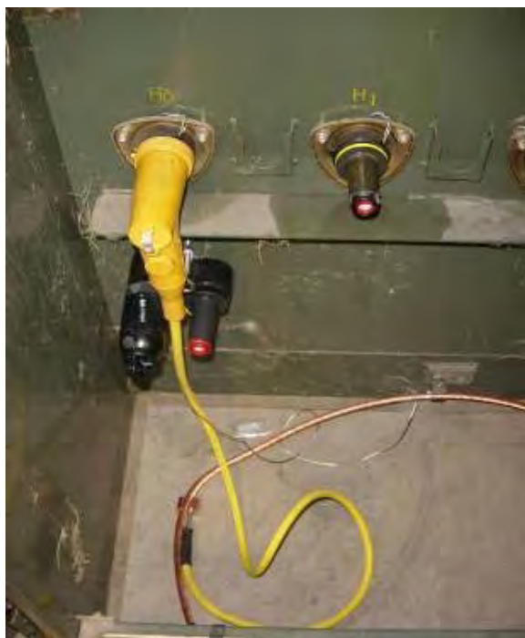
Figure #2 - Dead-Front Transformer, Dead-Front H0
