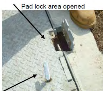
T wrench installed into hatch lock opener, if wrench is missing a large flathead screw driver can be used.
