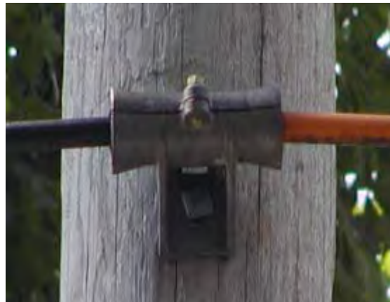
ADSS Rubber Clamp Insert and Metal Clamp
