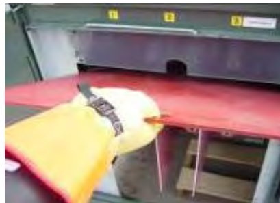
Switch compartment insert/remove barrier
