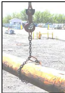
Examples of Correct use of Rigging
