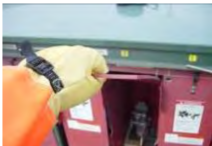
Fuse compartment insert/remove barrier
