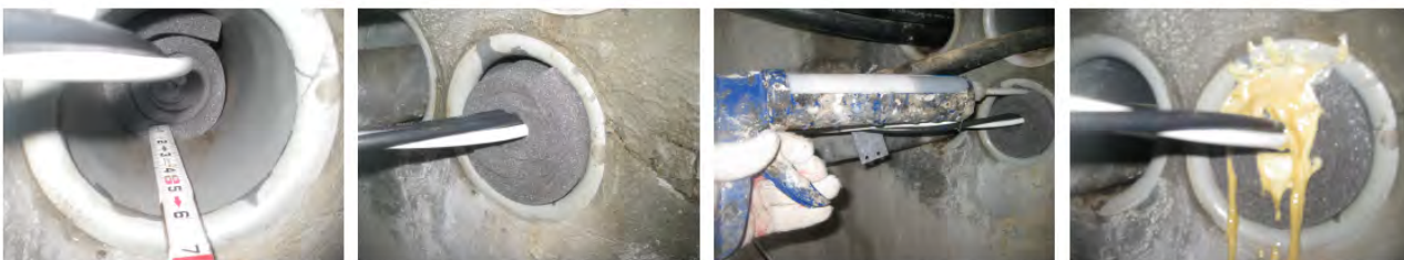
Water stop sealant installation
