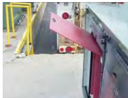
Switch compartment barrier fully inserted
